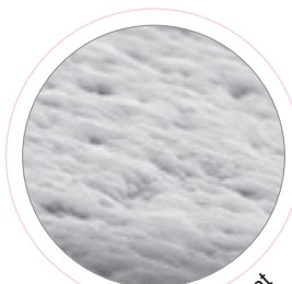
After surface treatment
